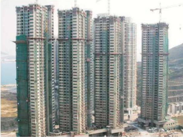
Tiu Keng Leng Station High Rise Building by Able
