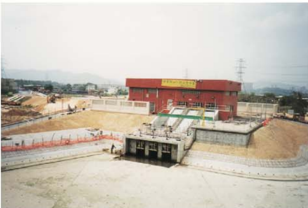
Pok Wai Flood Protection Works by Excel
